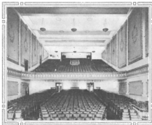
UNDER THE BALCONY DIRECT LIGHTING IS STILL USED IN THE PLAZA THEATER. Note the difference between this part of the interior and the remainder, which is illuminated by the indirect system.
