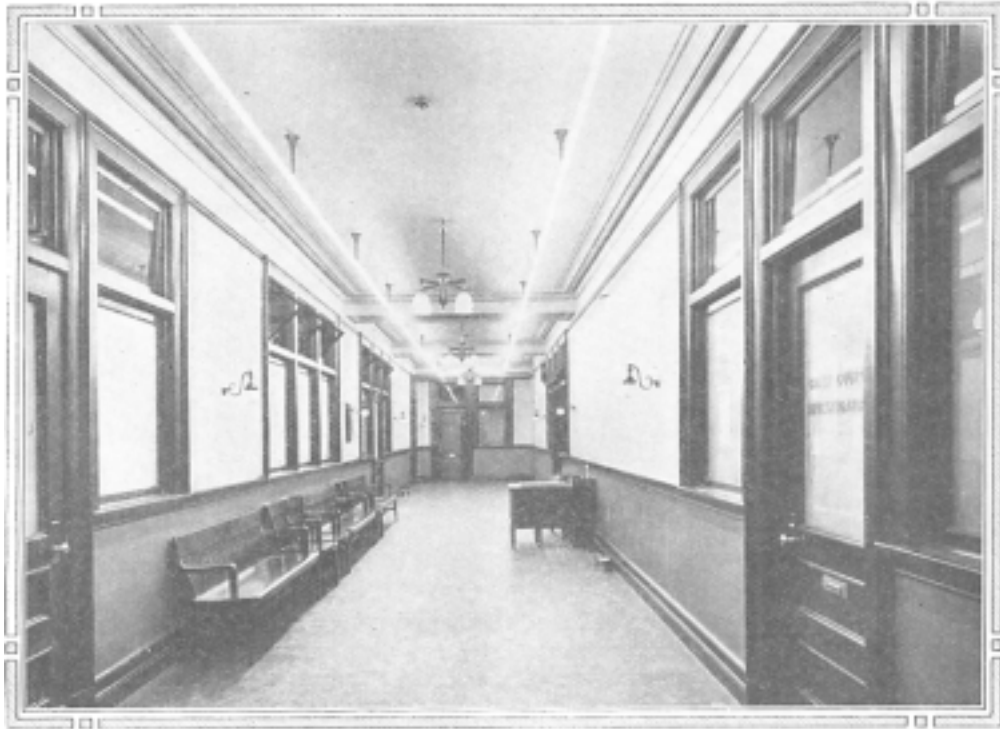
HALLWAY OF THE NEW PUBLIC SERVICE BUILDING, NEWARK, N. J., ILLUMINATED BY MOORE TUBES.
