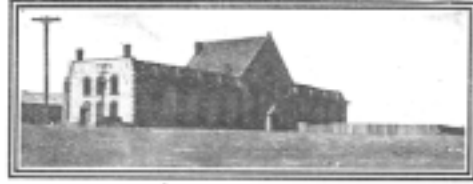
ABANDONED PENITENTIARY AT LARAMIE, WYO., WHERE GOVERNMENT SHEEP BREEDING IS BEING CARRIED ON.
