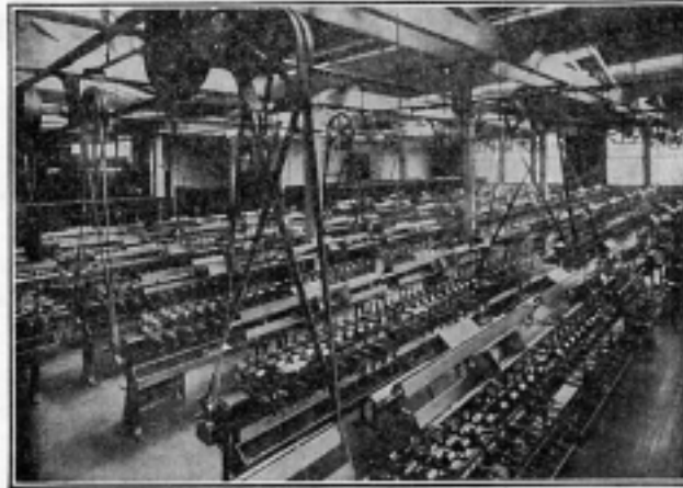
RECENT INSTALLATION OF "UNIVERSAL" FILLING WINDERS
